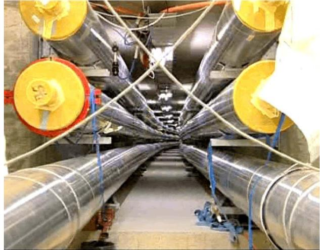
Fig. 4: Pulling the GIL into the tunnel
