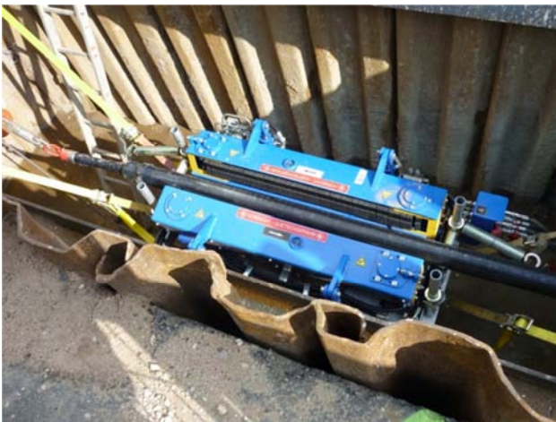
Figure 4: Hydraulic cable pushing device
