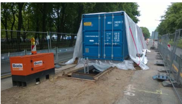
Figure 5: Joint pit in the middle of a street
