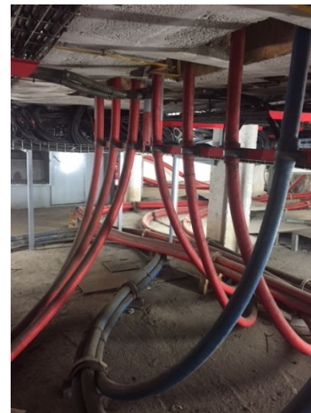
Fig. 1: Substation cable arrangement
