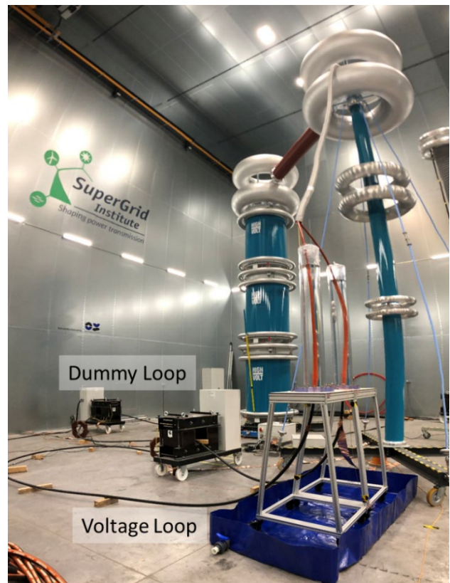
Figure 1: Characterized cable sample.
