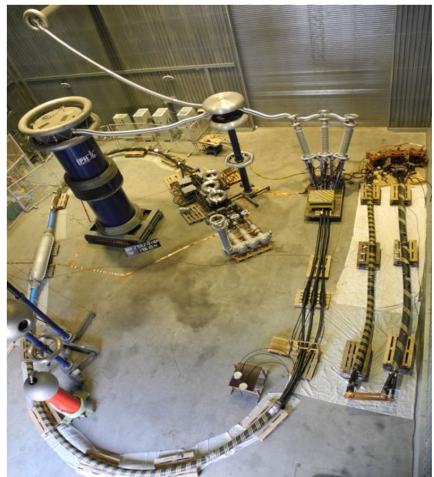
Fig. 1. Example of 3 phase AC submarine cable testing.
