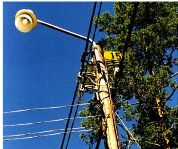
Fig.2. Joint installation between 24 kV, 1 kV, electric light and telecom cables
