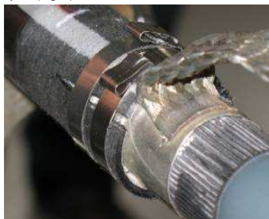
Fig. 3: Screen plate installed on the cable
