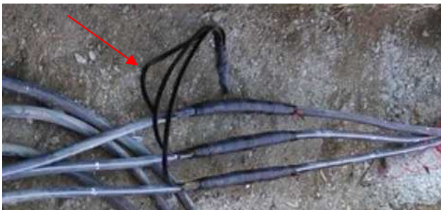
Fig. 1: Interconnection of the screens
