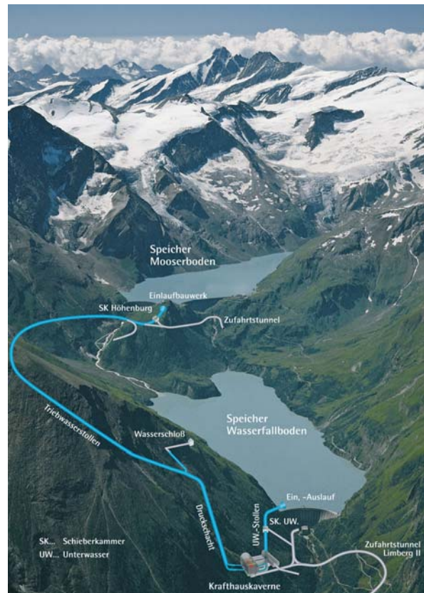
Figure 1: Photo-mounting of pumped-storage plant project Limberg II
