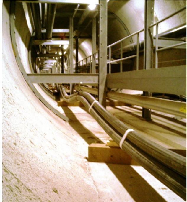
Figure 1: An orderly multi-purpose tunnel interior with HV cables and different pipes for transporting liquids and gasses.
