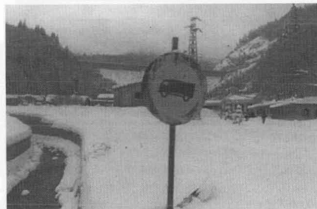
View of lower barrage
