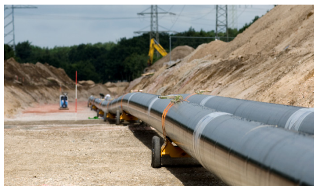
Fig. 1: Principle of a direct buried GIL during installation in the trench
