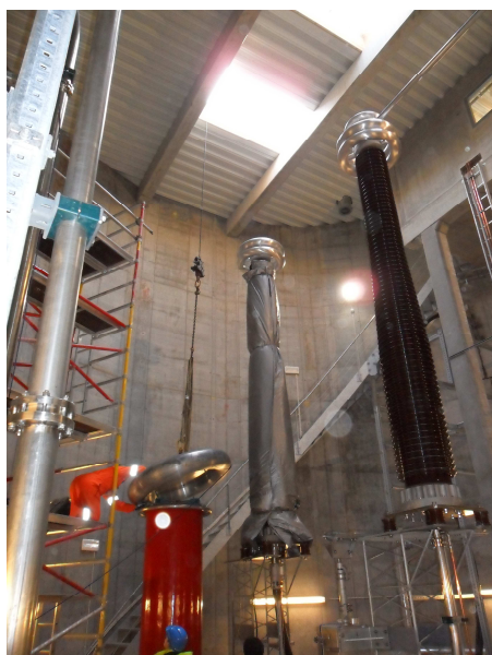
Fig. 3: Indoor air insulated terminations for the Kontek connection between Denmark and Germany.
