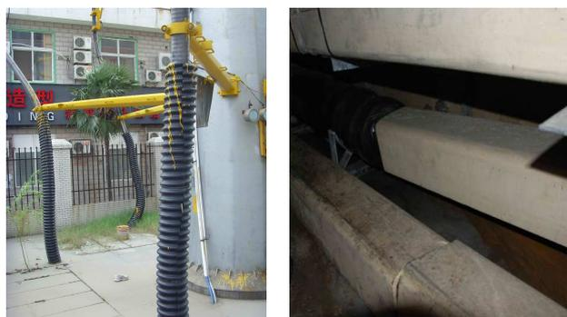
(a) Cable in vertical protect tube (b) Single cable in fire-proof box
