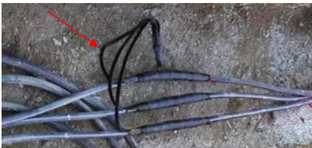
Fig. 1: Interconnection of the screens
