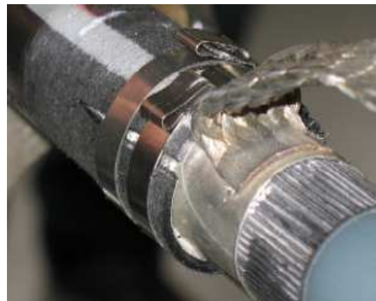
Fig. 3: Screen plate installed on the cable
