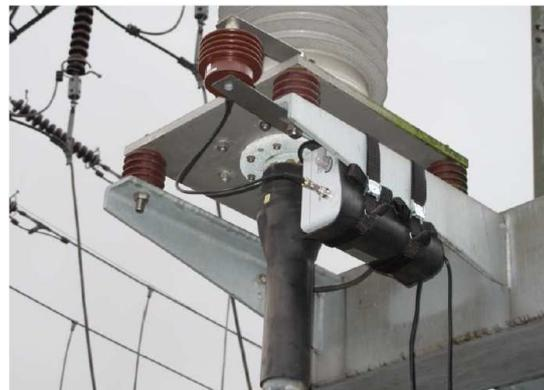
Fig. 1: Installed sensor and pre-amplifier.
