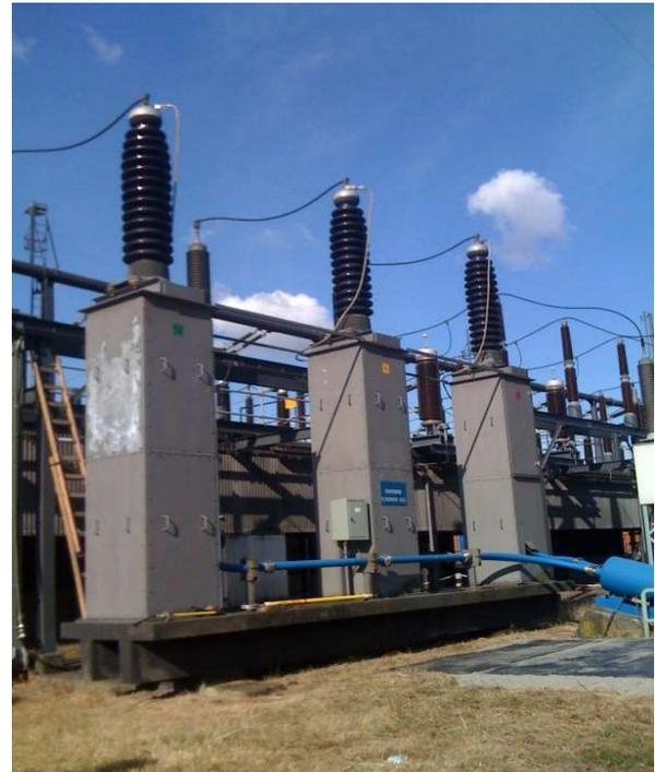
**Fig 1: Service-aged HV (150 kV) gas pressurized power cable.**
