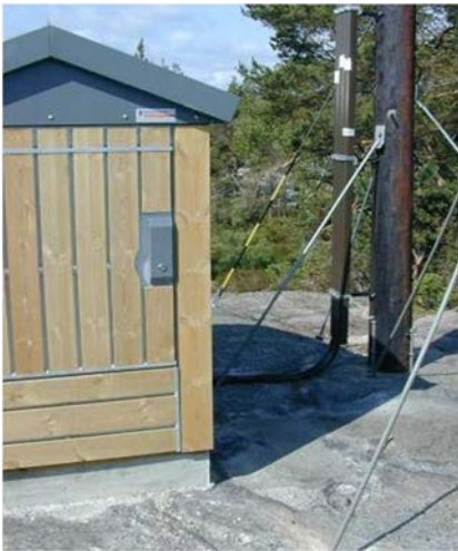
Fig 5-6 Cable from air into a substation
