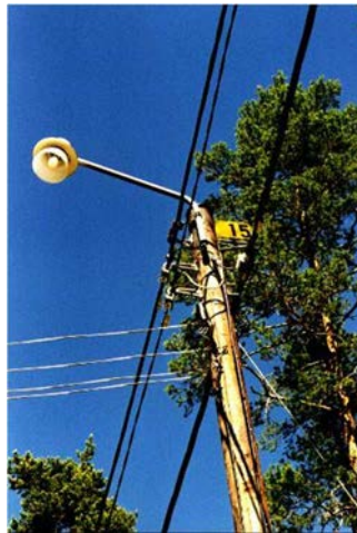
Fig 3 Joint installation
