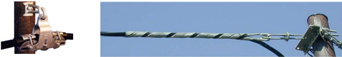
Fig 1 Cable suspension clamp and dead-end fixing helical
