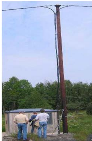
Fig 5-6 Cable from air into a substation
