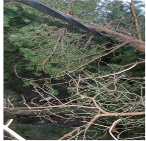
Fig 3 Trees on live cable after storm
