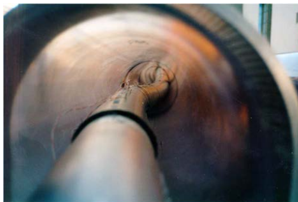
Fig. 1: Snaked cable into a pipe.
