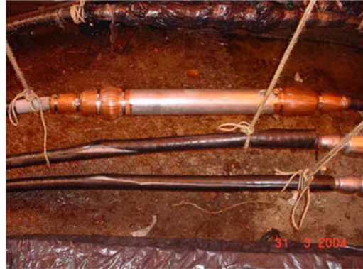
FIG - 3b Overlook of complete joint
