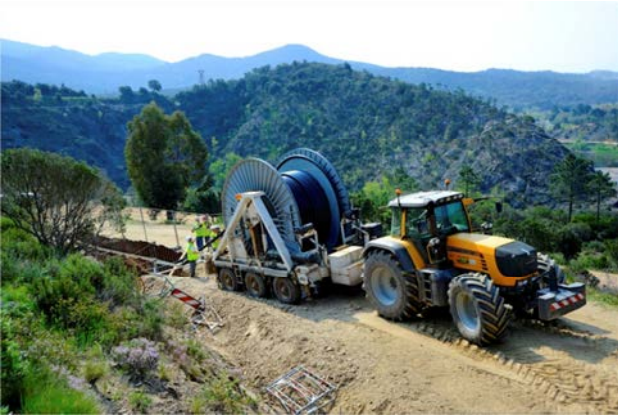
Figure 6: example of XLPE cable installation.
