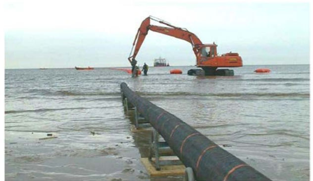
Figure 8: example of HVDC interconnection cable installation
