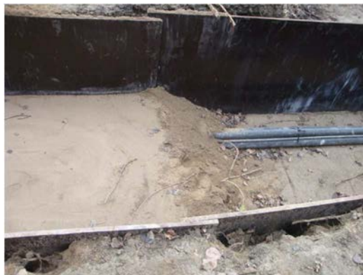
Figure 1: On site investigation of thermal backfills
