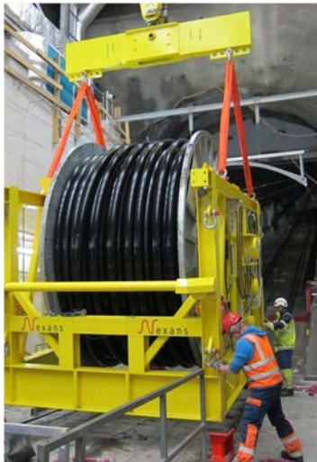
Fig.1a Loading of the laying bench on the cable car lorry
