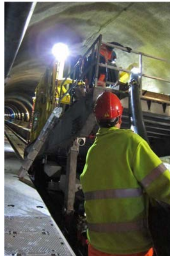
Fig.1b 380kV cable installation in the tunnel
