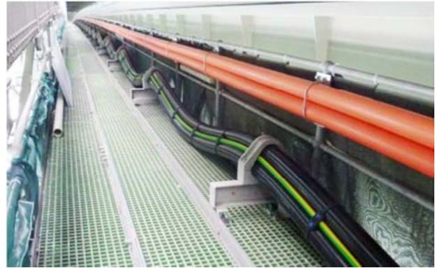
Fig. 9: Waved cables on Auckland Harbour Bridge
