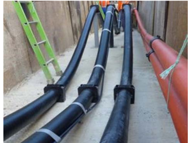
Fig. 3: Locking waves in a joint bay before backfill
