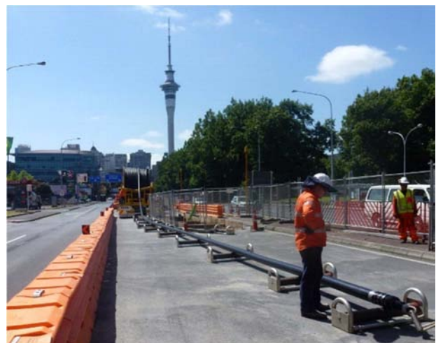
Fig. 10: Pulling cable into ducts near CBD
