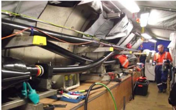
Fig. 15. Tunnel joint bay during construction
