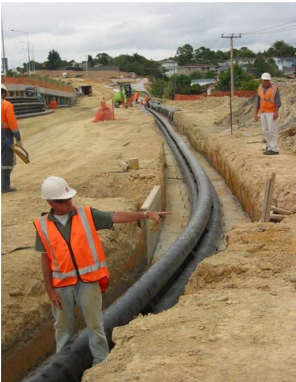
Fig. 2: Ducts installed under busway route
