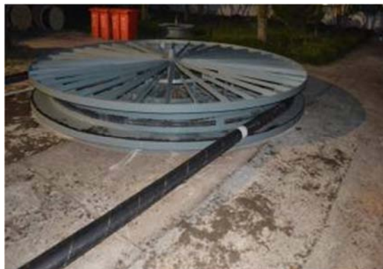
Fig.11 Bending tensile test site picture
