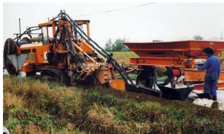
Mechanical laying in rural area
