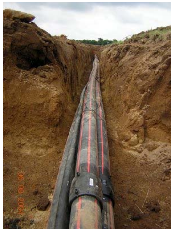
HDPE ducts, directly buried
