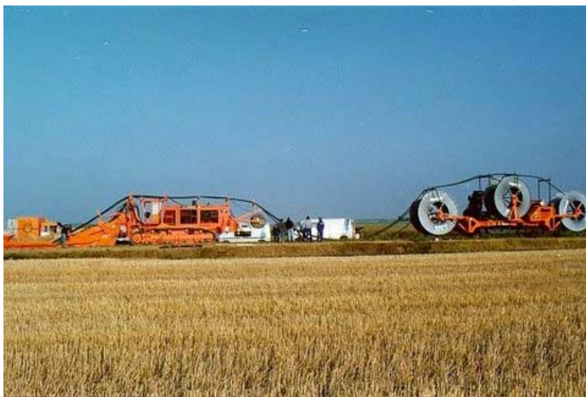
Mechanical laying in rural area
