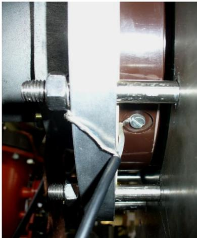
**Figure 12: Connection of a coaxial cable to the voltage sensor inside the bushing**
