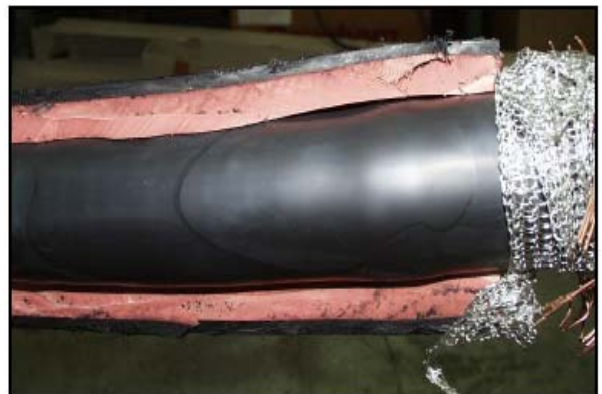
Figure 10: Gap between field stress tube and insulation tube due to incomplete shrinking
