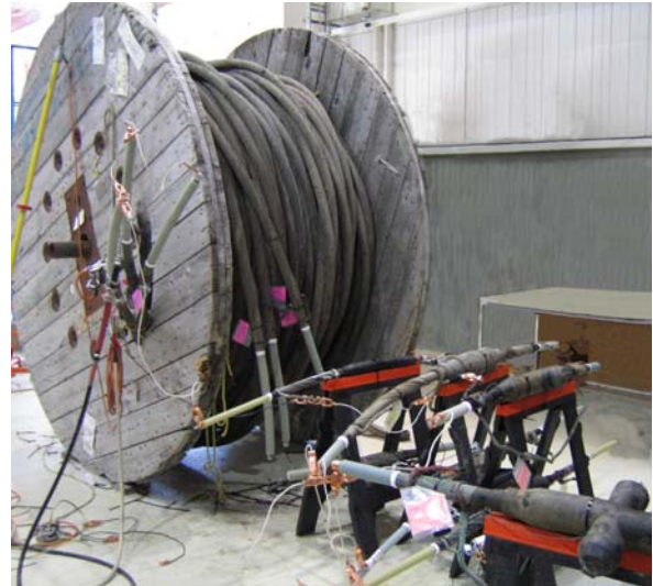
Figure 13: Set-up of cables and joints used for the line simulation measurements
