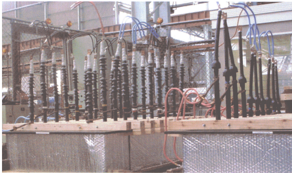
Figure 2: Water bath tanks in Test bay at the Ergon Energy facility
