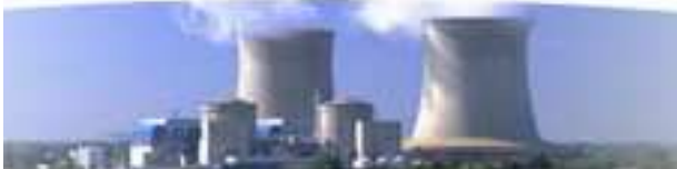
Figure 1: Cables in nuclear power plants may be exposed to irradiation.
