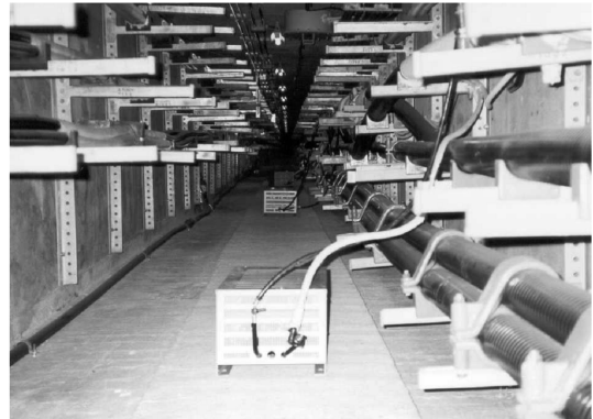
Figure 5: Sheath current reduction device (resistor)
