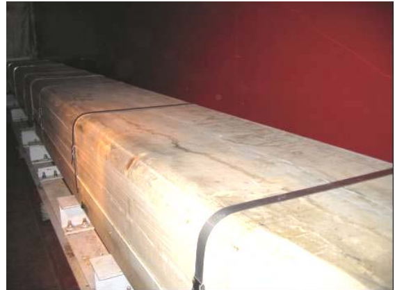
Figure 6: Example of fire prevention method for cable in tunnel by FRP trough
