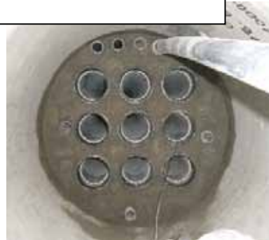
Pressure feed side
