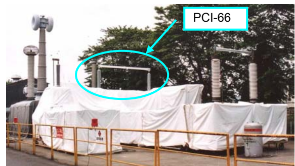
Figure 6: Long period heating-cycle voltage test
