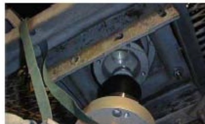
Figure 15: Assembly situation in the field
