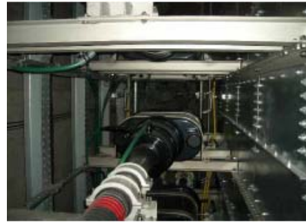
Fig.15. Installed YJB in the tunnel of TEPCO
