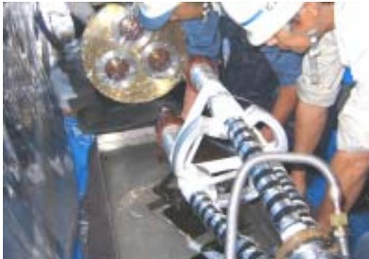
Figure-13. Jointing work in the imitated narrow manhole
