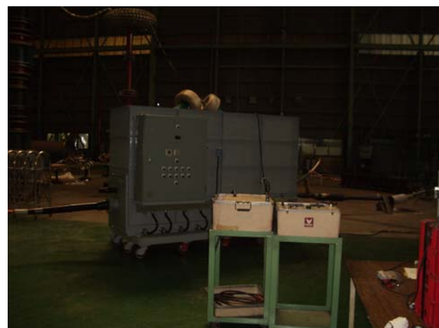
Figure 13. Test facility for outer protection test
