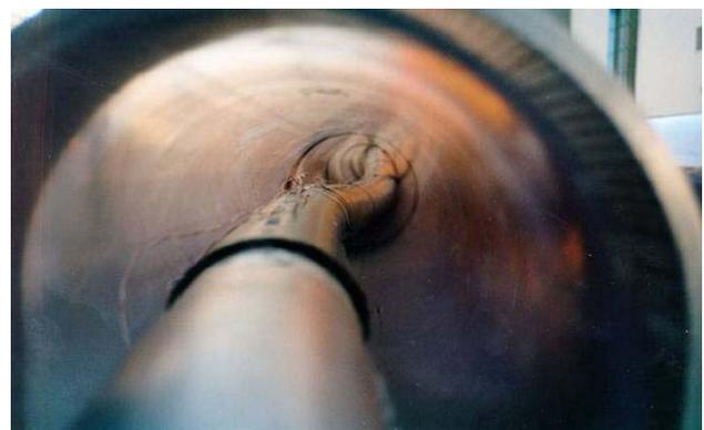
Figure 2: Snaking of a loaded HV cable inside a duct.
