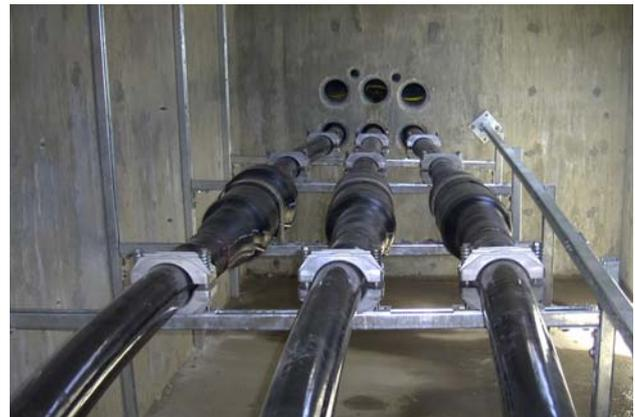
Figure 1: Rigid installation of Click-fit joints a manhole.
