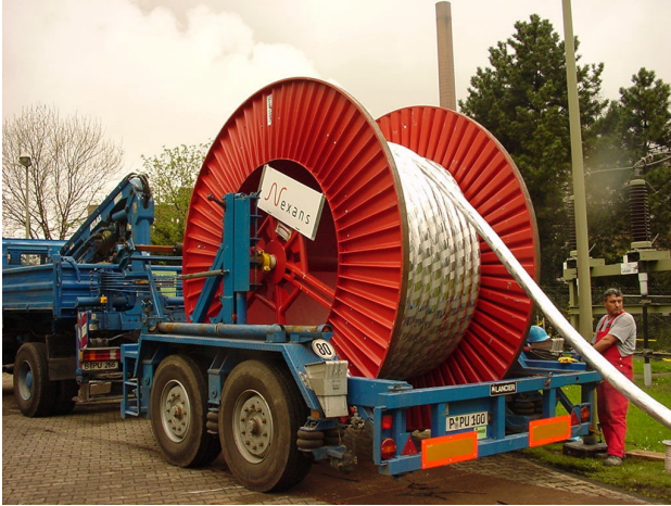
Figure 6: Laying of 110 kV three-core XLPE-cable
