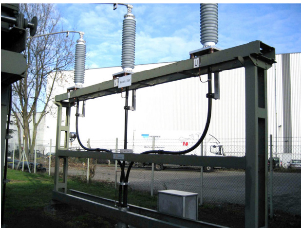
Figure 8: 123 kV outdoor terminations with composite insulator
