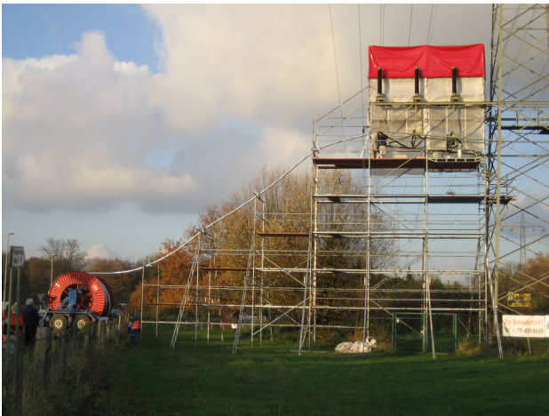
Figure 7: Cable pulling from the tower
