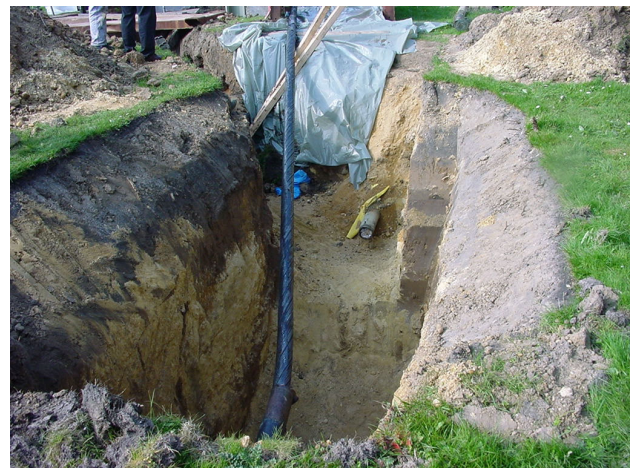
Figure 5: Recovering the old gas-pressure cable
