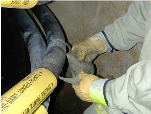
Figure 6: Measuring bending radius during inspection
