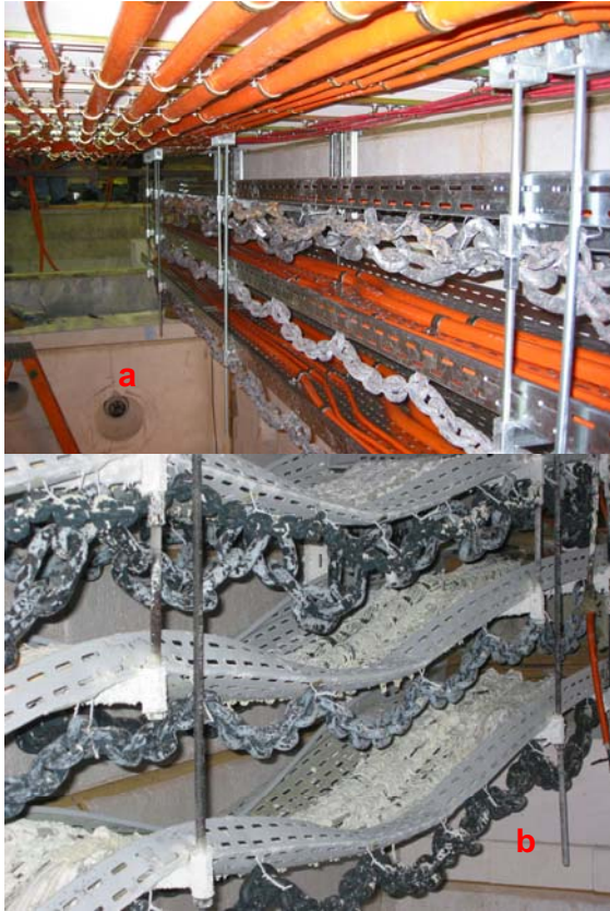
Picture 9 a&b: DIN 4102 part 12 before and after 90min in fire
