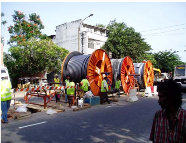
Photo 6: Cable drums in position, ready for cable installation.
