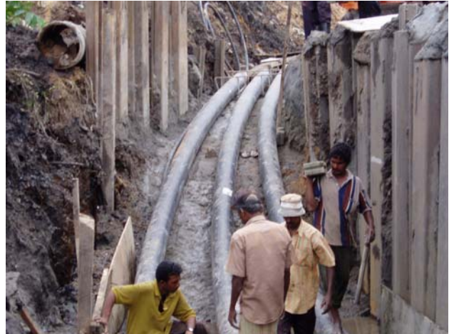
Photo 3: Installation in Marshy land
