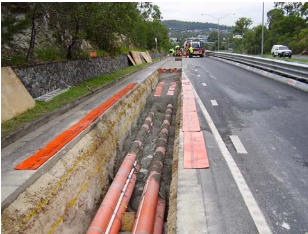
Photo 9: Backfilling of cable trenches.
