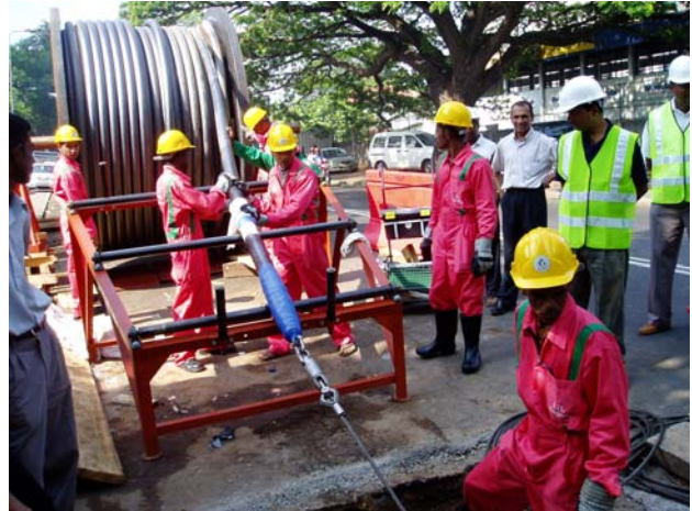
Photo 7: Cable installation in Colombo.
