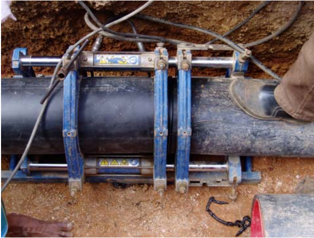
Photo 2: Jointing HDPE pipes
