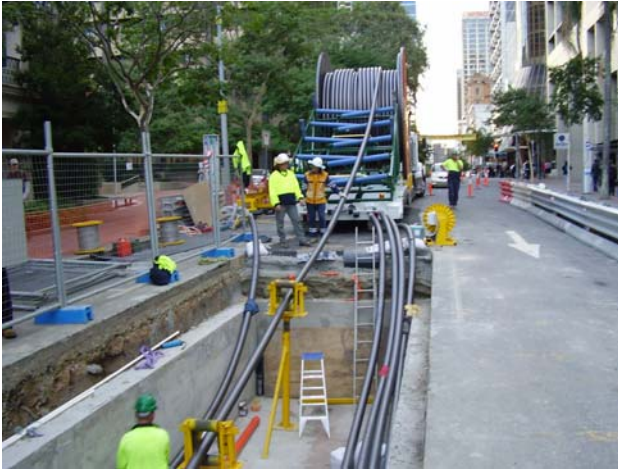
Photo 12: Cable Installation in Brisbane
