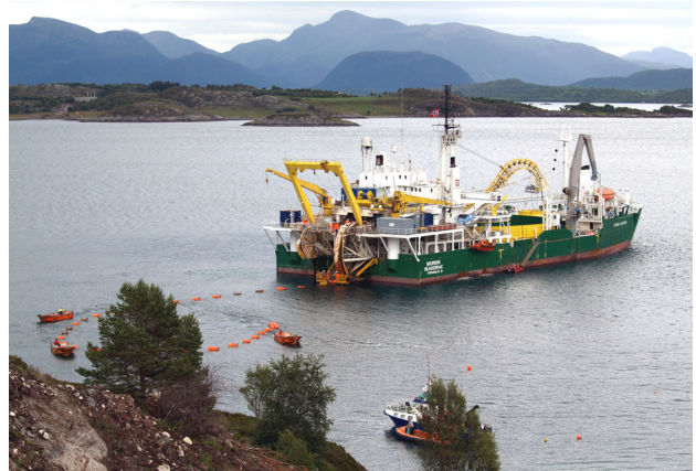
Figure 9. Cable laying with C/S Nexans Skagerrak.
