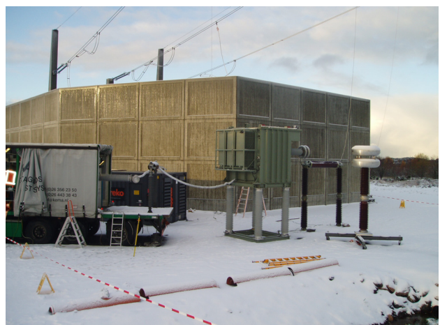
Figure 10. After installation test with transportable resonant test sets.
