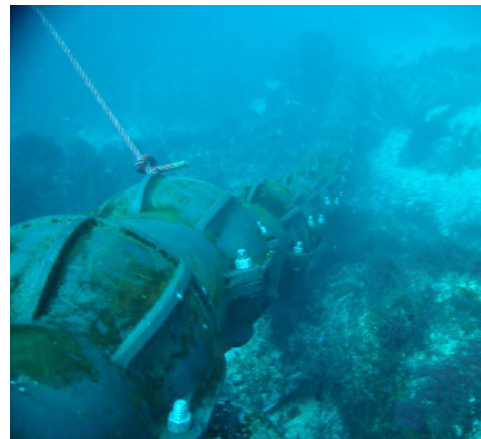
Figure 3 : Installation of cast iron shells
