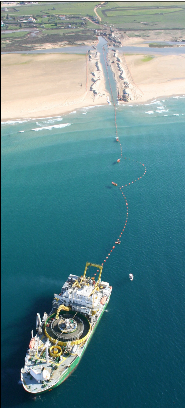
Figure 2 : Start of cable 7 laying in the Spanish coast
