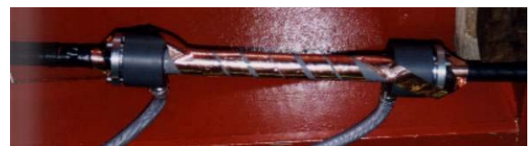
Figure 4 : The thermal diffuser (400 mm long) used to generate the thermal step from the outer screen.
