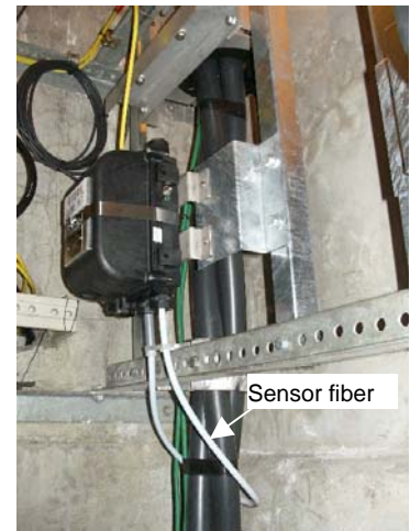
Fig.3.3 Practical application of the sensor to 66kV line
