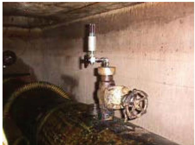
Figure 5: Sampling of a HPFF Cable by EDOSS
