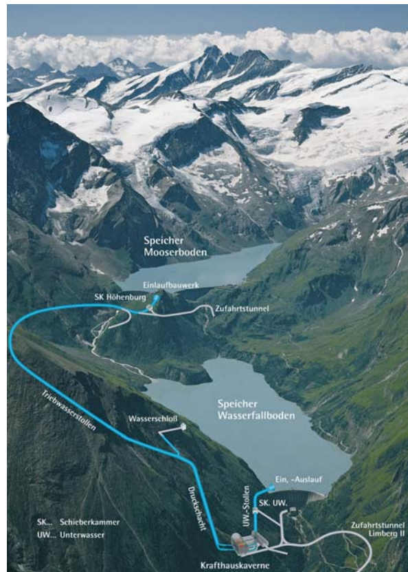
Figure 1: Photo-mounting of pumped-storage plant project Limberg II
