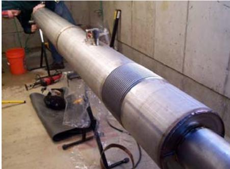
**Figure 8. Three-phase cable splice with housing**
