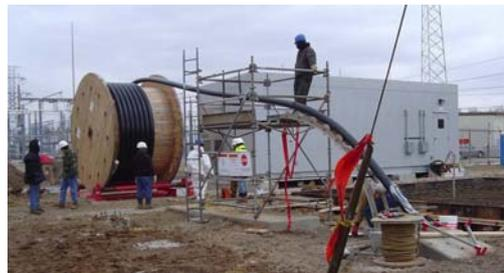
**Figure 6. Pulling of a cryostat section into a duct**
