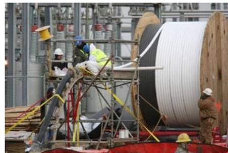
**Figure 7. Pulling of a cable section into a cryostat**
