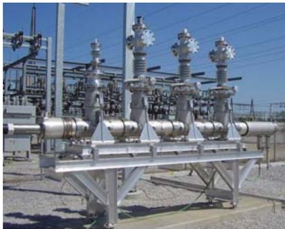
**Figure 9. Three-phase cable termination**
